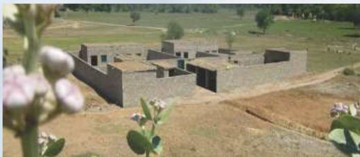
Shelter Homes for Flood Affectees in District Charsadda
